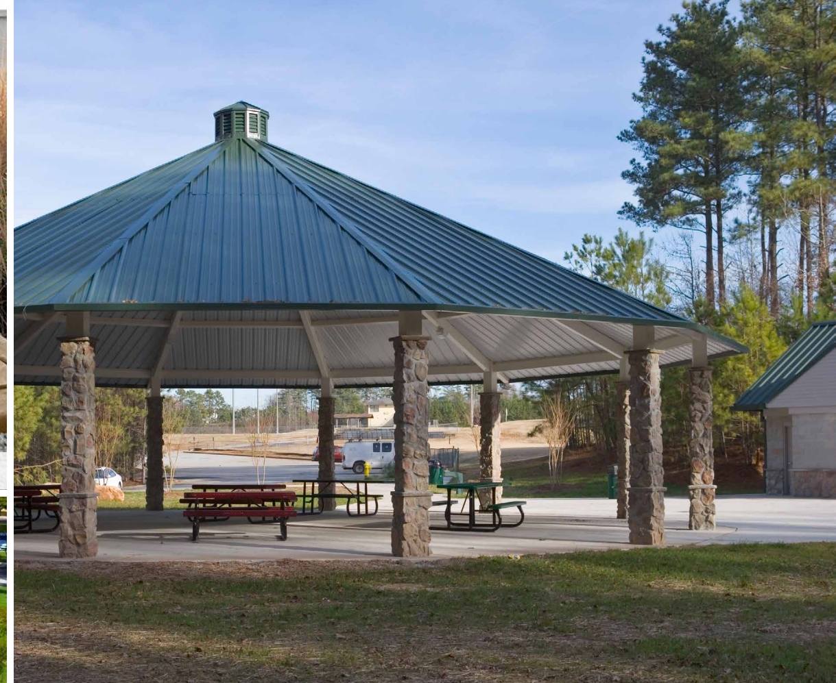
Wade Walker Community Park Pavilion, Atlanta, GA
