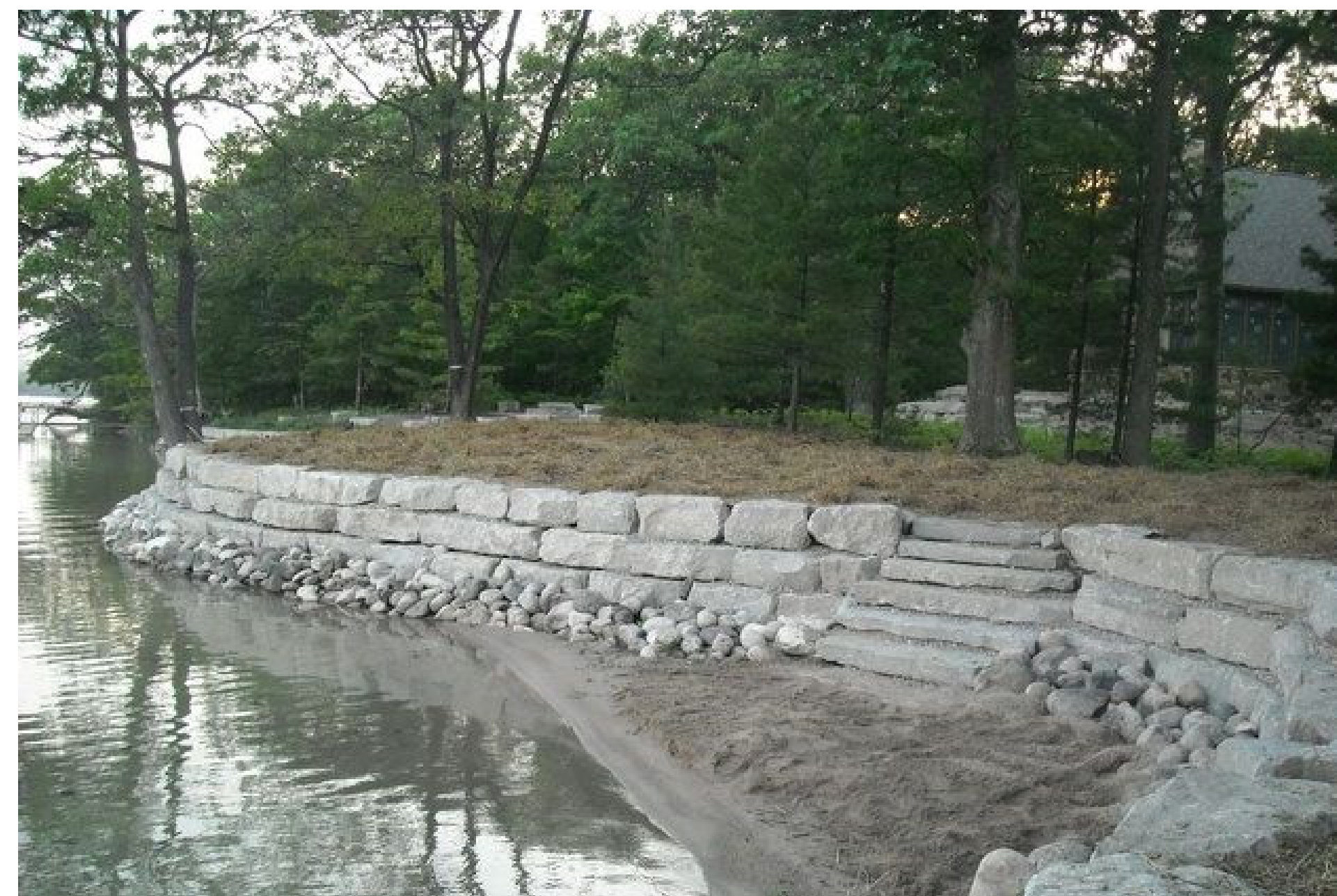
Armourstone Retaining Wall
