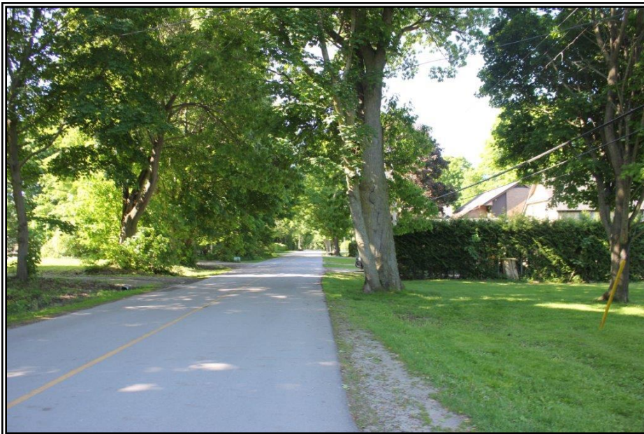
Streetscape of Morrison Avenue Looking Southerly
