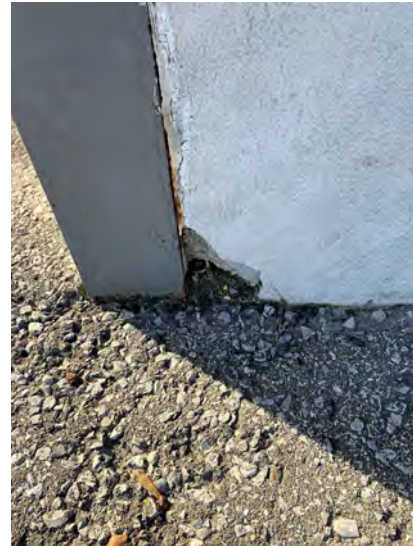
Photo 36 - South Elevation Opening
